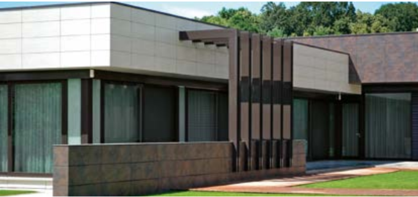
Private villa, Romania / Architect: Victor Gota / Year: 2016
