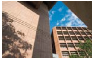
Lee Shan Building, Hong Kong, China
